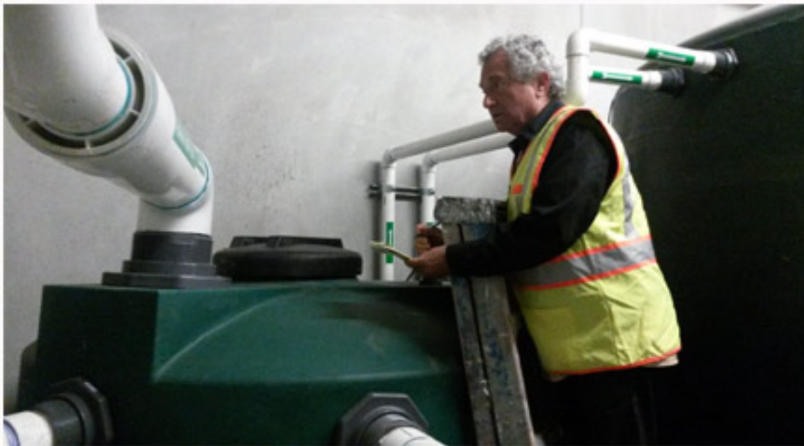
Bobby inspecting the tanks after their installation
