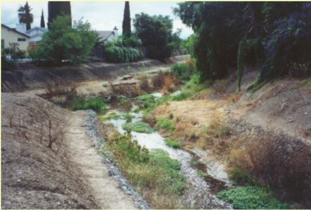
The creek before construction
